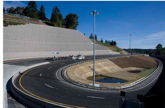
To create space for the new entrance, crews removed nearly 360,000 cubic yards of soil and built the tallest soil nail retaining wall in Washington State. The wall measures 90 feet tall and nearly 600 feet long. The new ramp to the joint campus was opened in September 2009 ahead of a challenging schedule.
