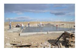
wind power by 2013. Construction began during the summer of 2009, and due to the importance of the project, it was fast-tracked to completion in just 12 weeks. WSI provided the construction layout of footings for all of the electrical structures and relay house, as well as the location of all underground utilities and site grading. WSI also worked directly with BPA surveyors in establishing and maintaining project survey control.
